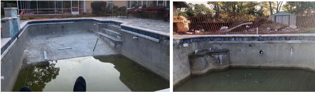
Photos of the unfinished pool.
